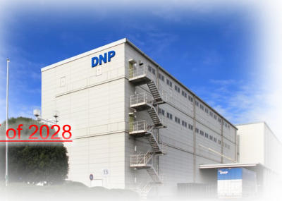
Kuki Plant (Saitama Prefecture)
