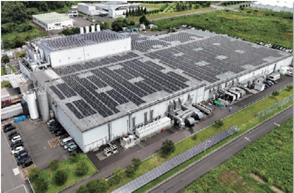
Solar power generation system at the Izumizaki Plant
