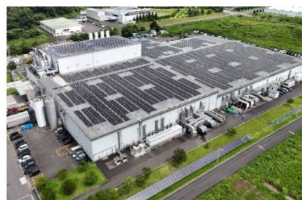
Solar power generation equipment at the Izumizaki Plant
