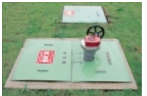
Tokyo Plant, The Inctec Inc. Emergency Shutdown Valve
