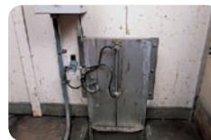
Wastewater conduit shutter Kyoto Plant, Dai Nippon Printing Technopack Kansai Co., Ltd.
