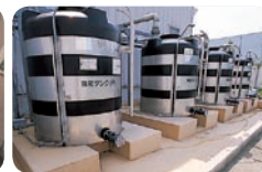
Leakage retaining walls Ushiku Plant, DNP Data Techno Co., Ltd.
