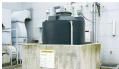
Leakage retaining wall/Utsunomiya Plant, DNP Graphica
