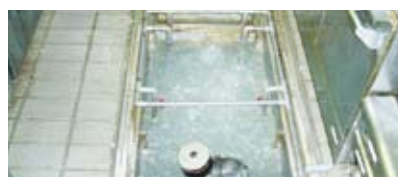
Grease trap processing equipment/Enokicho Plant, Commercial Printing Operations
