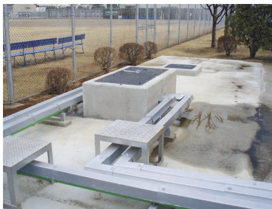
Holding tank replacement (two-tier construction, anti-leak sensors installed)
