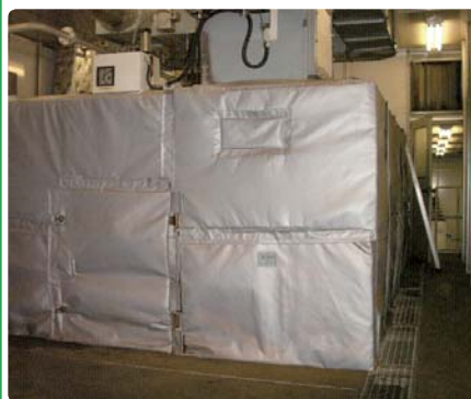
Jacket insulation on deodorizer
